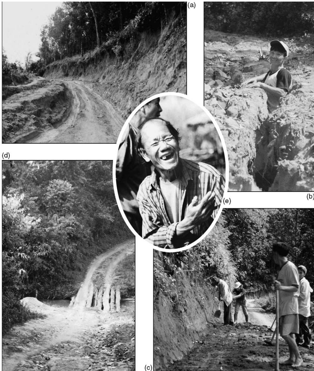
Fig. 1. Road features in northern Thailand: (a) unpaved mountain road near Pang Khum, an annual source of sediment to the stream system; (b) deep incision on the upper PKEW road (ca. 1998); (c) Pang Khum villagers repairing road ruts by filling with material taken from the cutslope; (d) typical low-water bridge where road runoff and sediment enters the stream; (e) Lisu man acknowledging that road impacts are no laughing matter.
