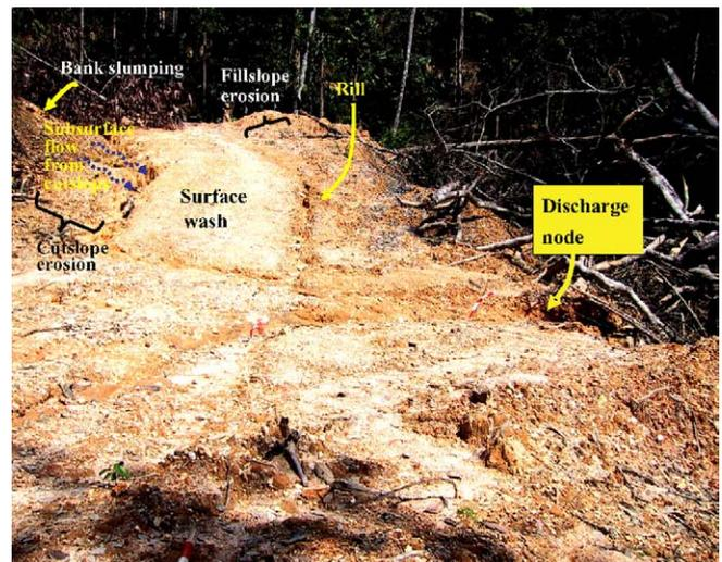
Fig. 5. Rill and gully erosion on a logging road in central Malaysia. Erosion features indicated on the photograph converge at a discharge 'node' located at a topographic low point on the road. Water and sediment discharged at this node connect directly to a headwater stream.
