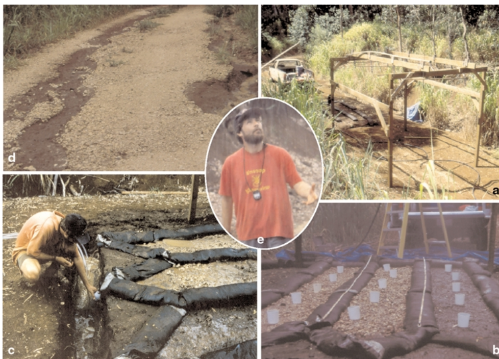
Figure 1. (a) The car-wash-type, low-energy simulator on the experimental road section at Schofield Barracks. (b) The three side-by-side treatment plots. (c) Runoff sample being collected during a simulated event. (d) Deep ruts formed on an adjacent road that has been surfaced with the coral-derived material tested herein. In panels (b) and (c), the treatments from left to right are 1xCoral, 2xCoral, and bare.
