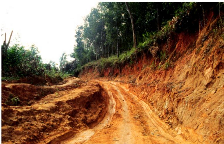
Figure 3. Surface lowering on the main road to Pang Khum. The  $>0.5$  m elevated bench on the left was the original road surface before the rainy season began four to six months earlier
